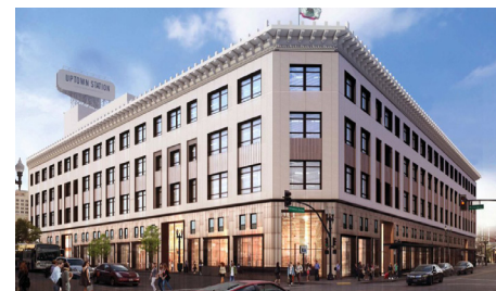
UPTOWN STATION, OAKLAND
